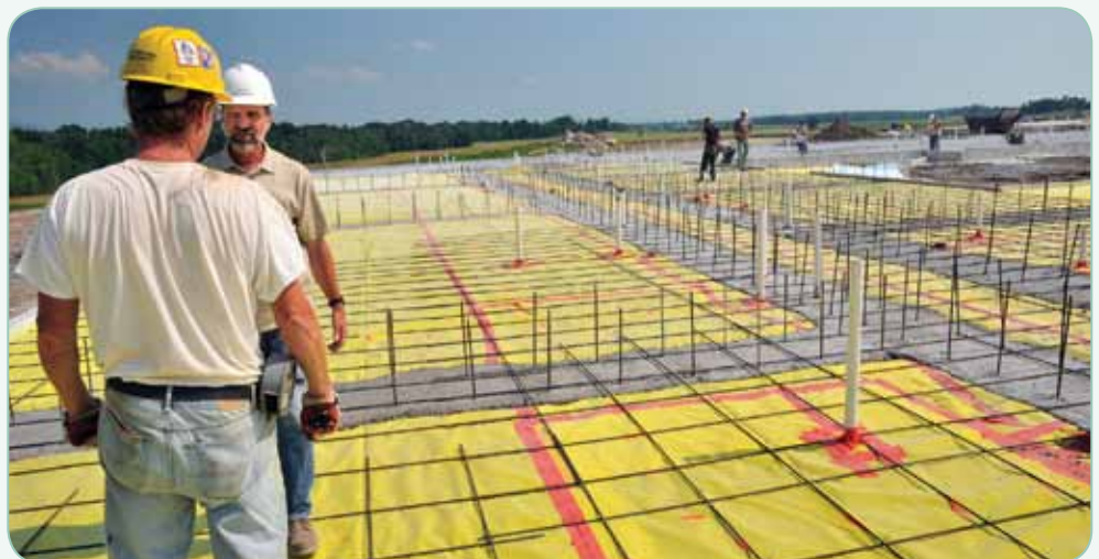
Construction crew preps Inn foundation for the pouring of the slab.
