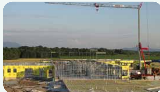
Walls start to go up on the Inn, August 4
